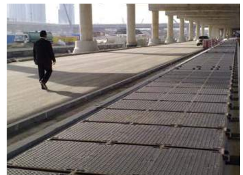
Continuous duct cover
