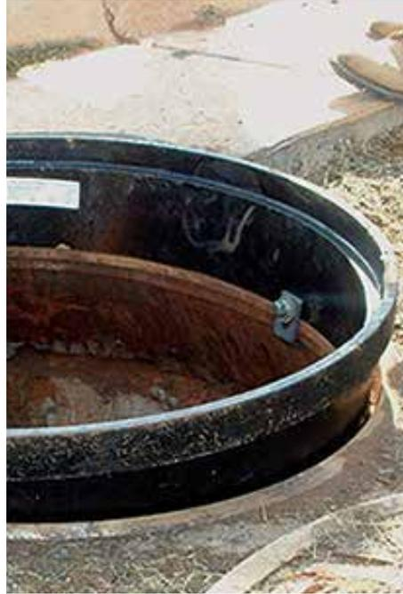
Riser rings are an adjustable solution to bring a manhole or catch basin to grade on your resurfacing projects. They are used in conjunction with a frame to increase its overall height. A typical application would be during pavement overlays.
