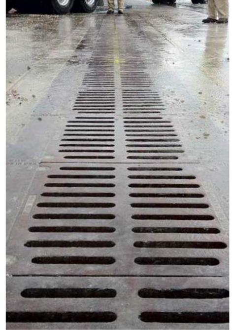
From pedestrian areas to airport loading ramps, EJ has the trench drainage solution to fit your application. With a grate that is designed to be supported on two sides, it is expandable and available in numerous widths.
