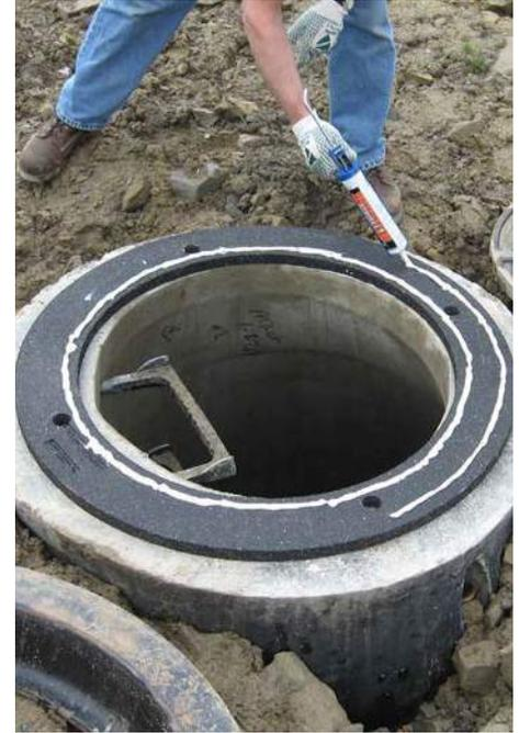
Maintain the integrity of your infrastructure by reducing traffic vibration damage. Adjust any manhole or catch basin to grade on your resurfacing projects, new installations, or rehabilitation work with INFRA-RISER® rubber composite adjustment risers.
