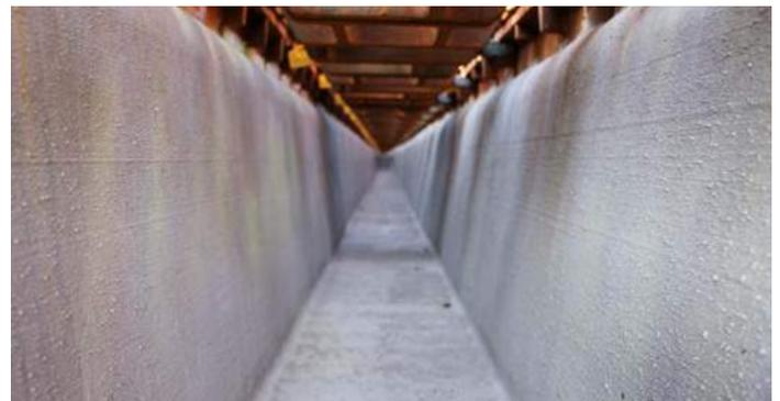
Designed to work with concrete trench forming systems that improve the speed of installation versus traditional installation. Using concrete, no liners are needed—eliminating combustible material in applications where fire suppression measures are needed.
