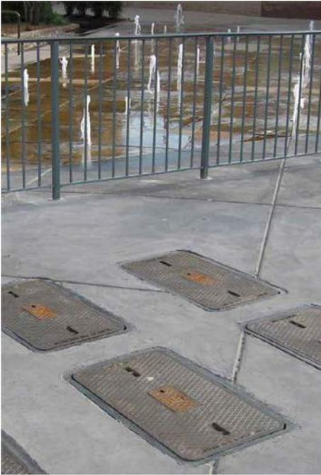
The meter box product is specifically intended to cover a water meter. It is typically large enough to allow for inspection and limited access, and is often intended for non-traffic situations.
