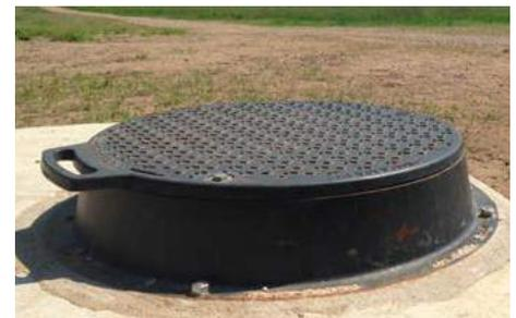
The surface of the cover extends slightly past the edge of the frame, and the neoprene gasket helps seal the unit against water infiltration. A watertight seal can be achieved with the four bolt design.
