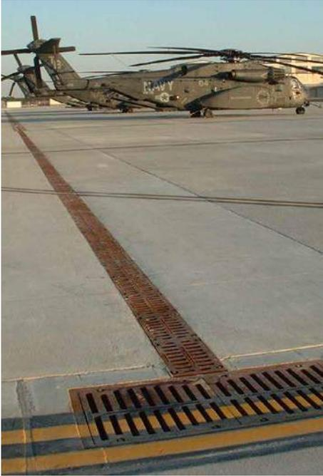
Environments that undergo excessive load conditions require construction castings specifically designed to meet or exceed heavy duty load rating standards. EJ offers many solutions for these types of applications.
