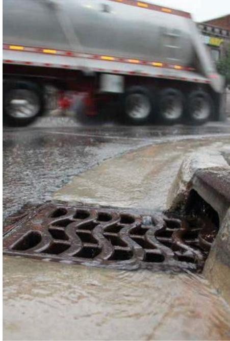
Drainage castings or grates are designed to accept water and can be round, square, or rectangular. They are typically sold with a frame, curb inlet frame, monument box, or bridge drain. Some markets call these slotted covers.
