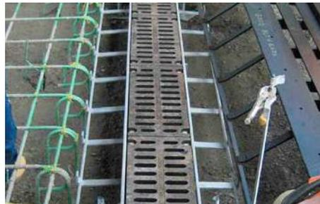
Build to any length of drainage required and incorporate cast iron trench or fabricated steel grates to meet your project needs.
